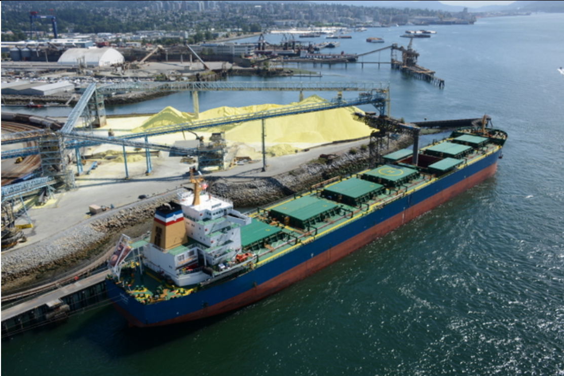
Photo bc17_br_00272: Example of Coastal Class 32; Permeable man-made structures. Vancouver Harbour.
