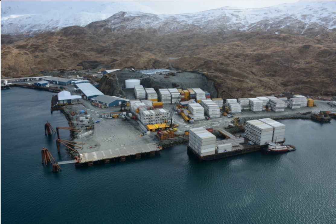
Photo ai16_ua_03348: Example of Coastal Class 32; Permeable man-made structures. Captains Bay, Unalaska Island.
