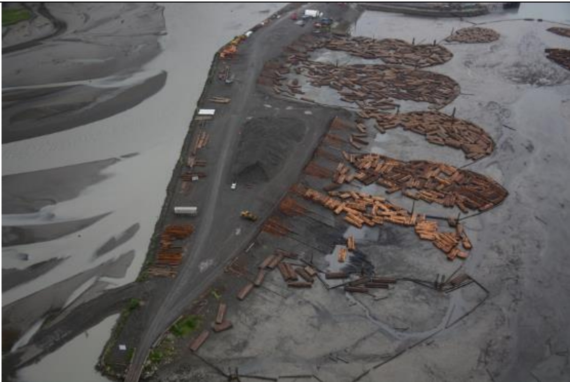
Photo bc15_sh_16416: Example of Coastal Class 32; Permeable man-made structures. Stewart, BC.
