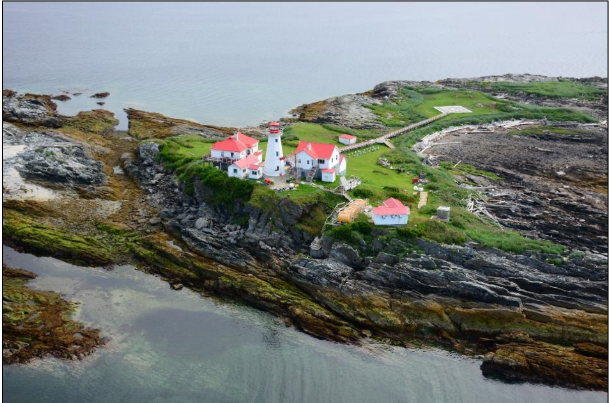
Green Island Lighthouse, Green Island
