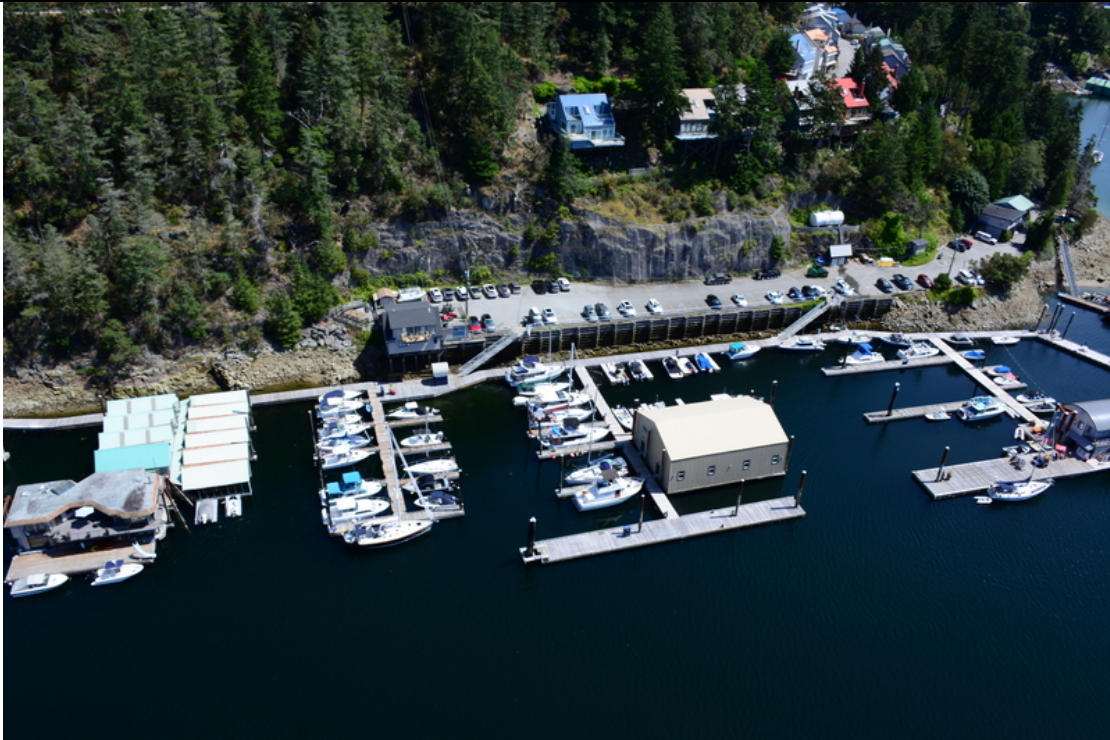
Photo bc20_sc_14094: Example of Coastal Class 32; Permeable man-made structures. Secret Cove.
